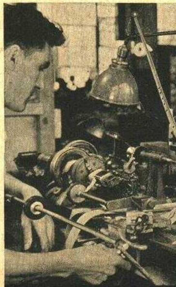
8 - WINDING POWER-TRANSFORMER COILS
