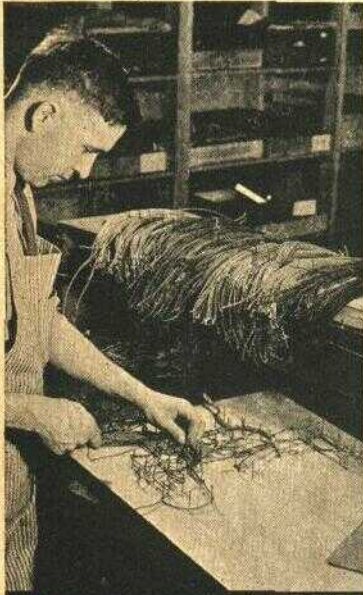
4 - FORMING MAIN WIRING CABLE
