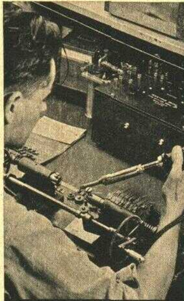
5 - WINDING ATTENUATOR RESISTANCES
